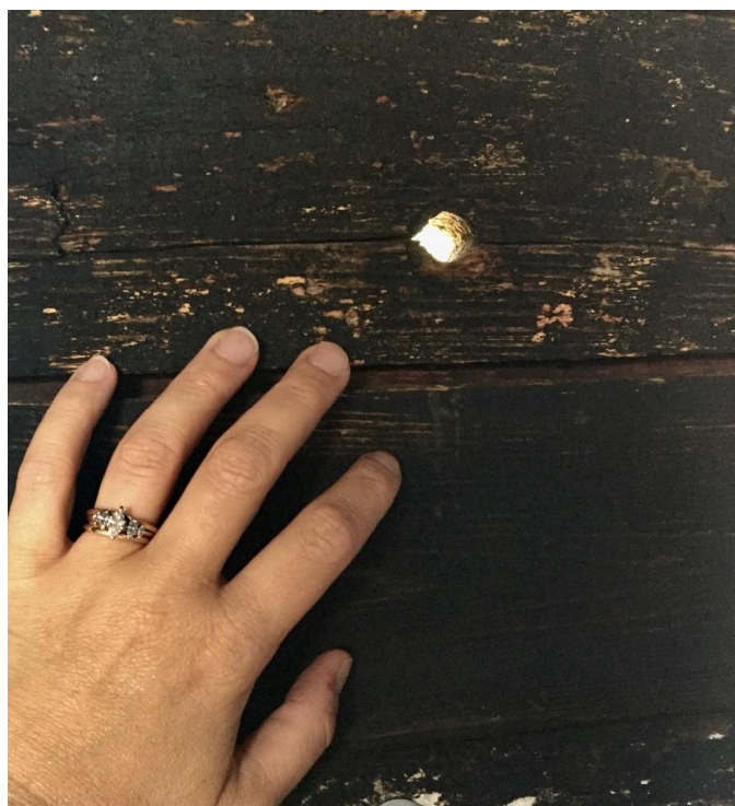
Inside of the boxcar, formally used to carry victims to prison camps, labor camps, or death camps. The boxcar had substantial wear and needed repair, but the walls were original.
